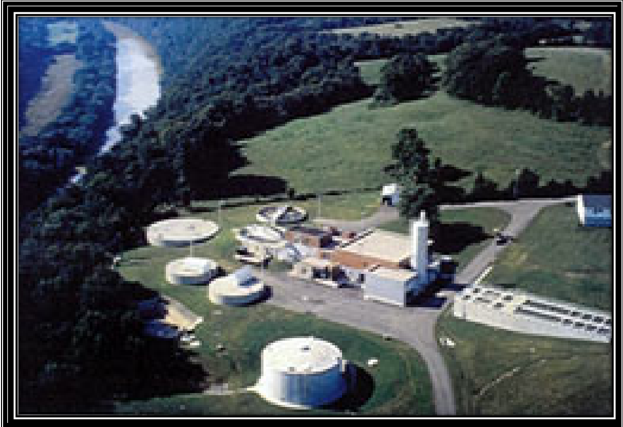
Figure 2 Nicholasville Water Treatment Plant
